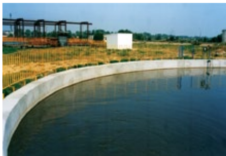
Waterproofing a sewage treatment plant, Bielsk Podlaski, Poland.
