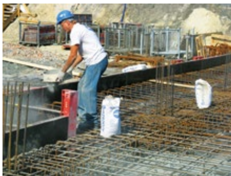
Waterproofing the bottom of a foundation slab, Katowice, Poland.
