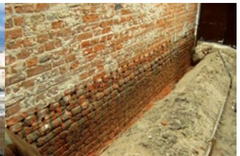
Restoration of vertical and horizontal waterproof protection, Białobrzegi, Poland.
