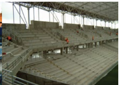
Waterproofing concrete elements on a stadium terrace, Kielce, Poland.
