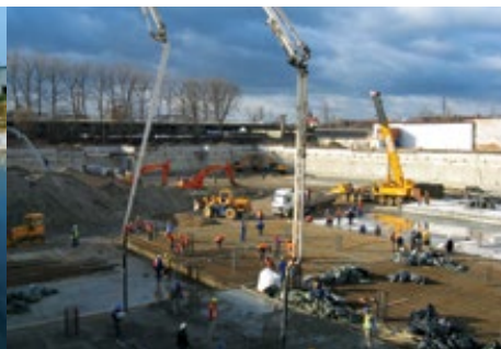
Waterproofing a foundation slab and slab-to-slurry wall joint, Kraków, Poland.
