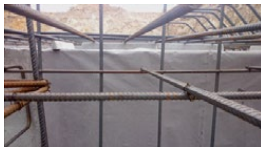
Photo. 2. Concrete being poured over a wall, with the surface covered with Penetrating Mat .
