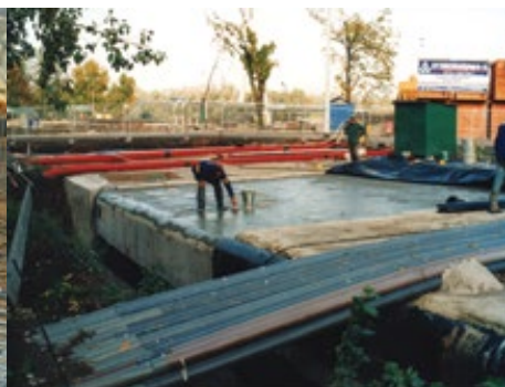
Waterproofing the top of the roof structure on Tunel Świętokrzyski, Warszawa, Poland.
