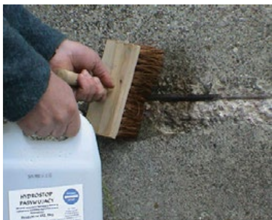
Fig. 1. Soaking concrete around a rod whose protective coating is not sufficient. After this procedure the surface will be reprofiled.
